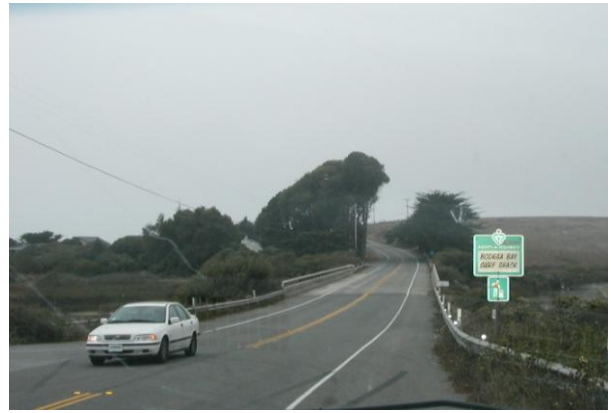
Highway 1 at Salmon Creek Bridge, looking north
