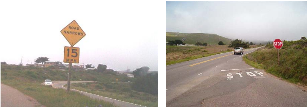
Highway 1 at Keefe Ave., looking north
